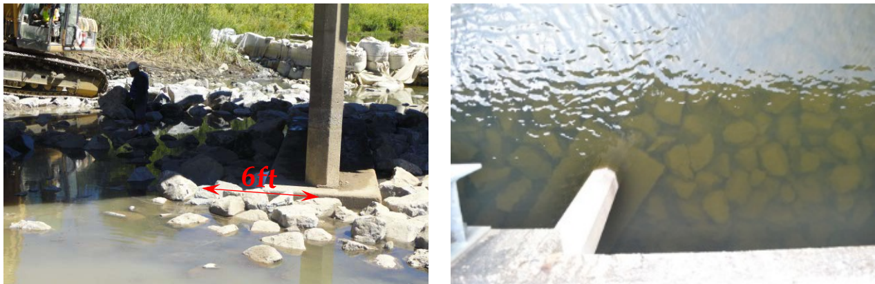
Figure 2.4: Pictures of riprap installation near Pier-3 during and after the construction
