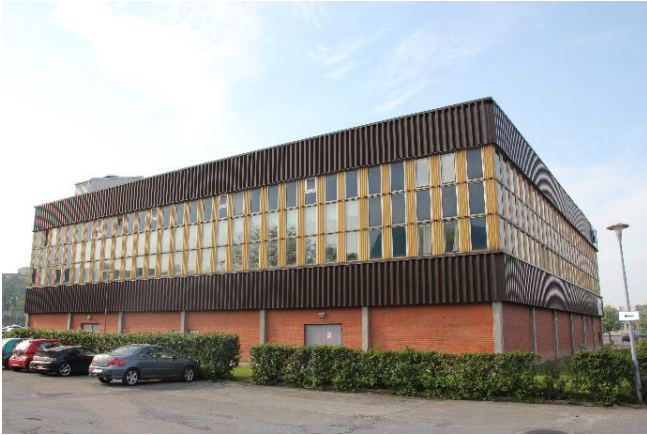
Fig.2: Gompute Data Center, Gothenburg (Sweden)
