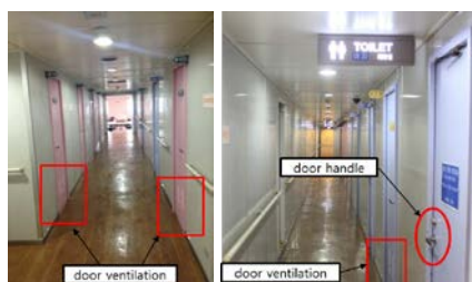
Fig.10: Door ventilation and general office door handle at door in cabin decks
